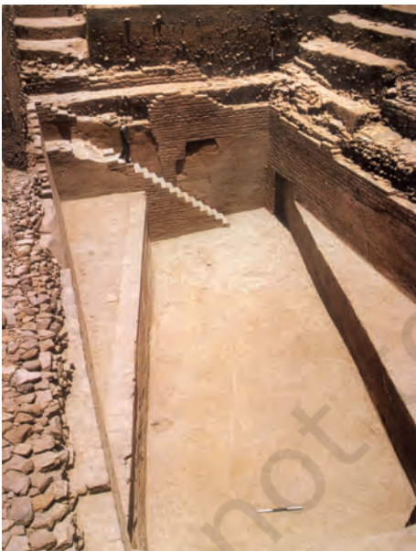
Fig. 1.5 Reservoir at Dholavira Note the masonry work.
